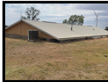
North side of house
